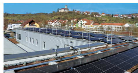
Solar panels at the MBO plant in Germany
