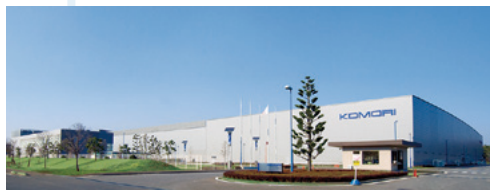
2009 3rd Phase Construction of Tsukuba Plant Completed
